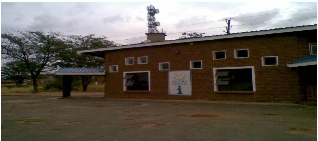
Figure 7.9: Main infrastructure of the Musina Municipality Tourism Info Centre. Source: Researcher, 2019
