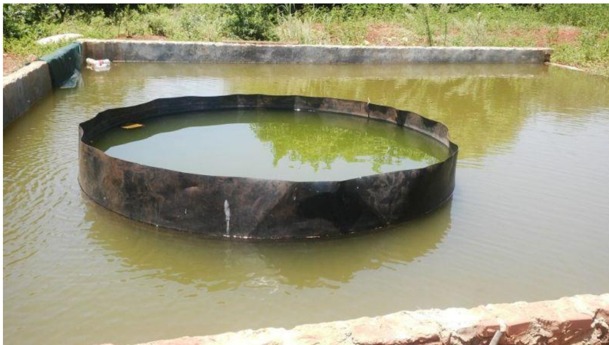
Figure 20: The concrete and plastic fish dam for Mr. Mufunwaini
