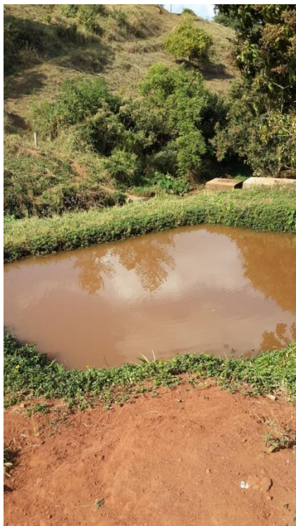
Figure 12: The earthen fish dam for Mr. Tshivhase
