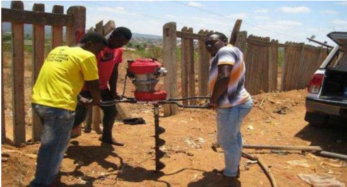
Plate 3.2: Installation process of the monitoring probes in Thohoyandou landfill
