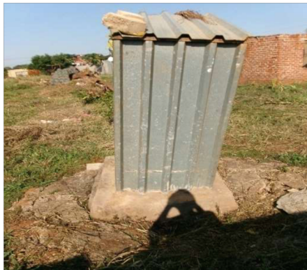
Figure 4.5: Pit latrine used by one of the respondents.
