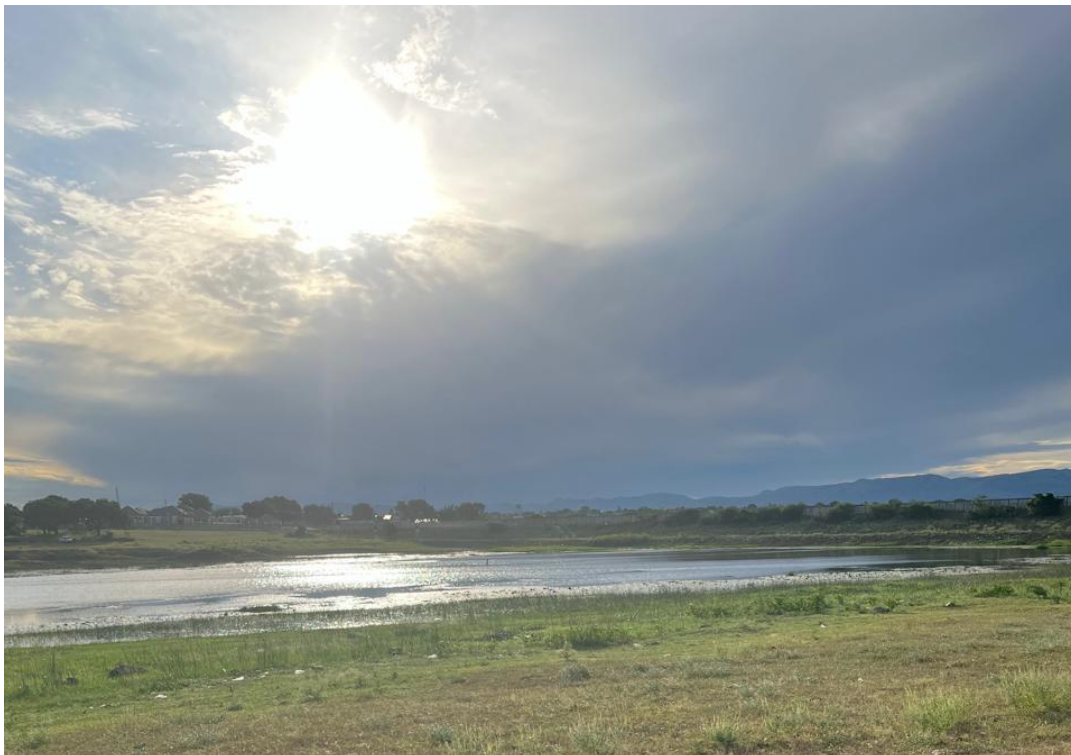
Plate 5.6: Driekoppies Dam Source: Author (2024)
