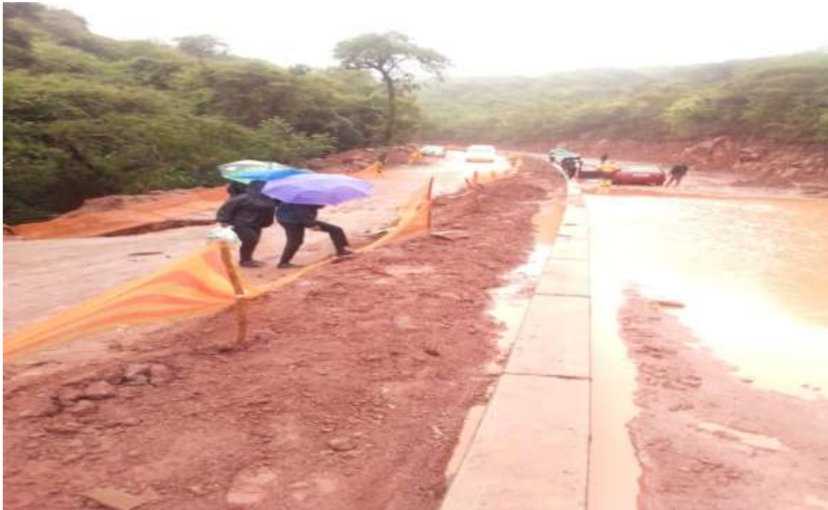
Figure 9: Poor road infrastructure due to extreme weather conditions
