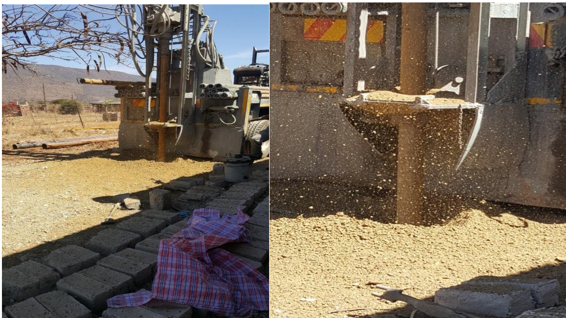
Figure 3.1: Drilling operation at Siloam Village
