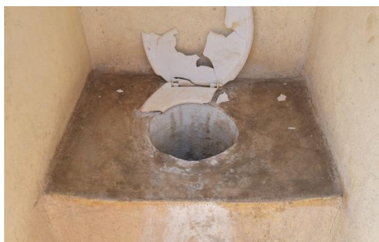
Figure 2.3: Pit latrine toilet ( https://www.dailymaverick.co.za/article/2018-07-31-finally-urgent-new-plan-to-eradicate-pit-toilets-at-schools-to-be-unveiled/ )[Accessed August 2018]
