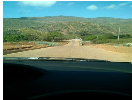
Fig: 2.4.B. Recently completed tarred road
