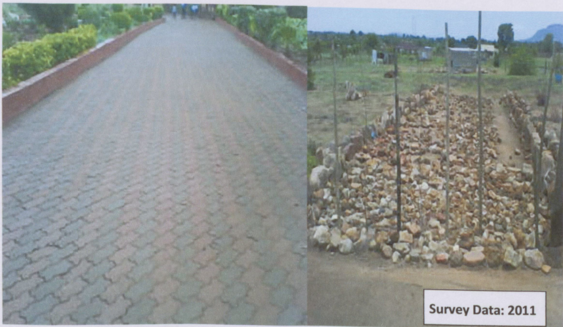
Picture 4.8 Paved surfaces in Thohoyandou Township
