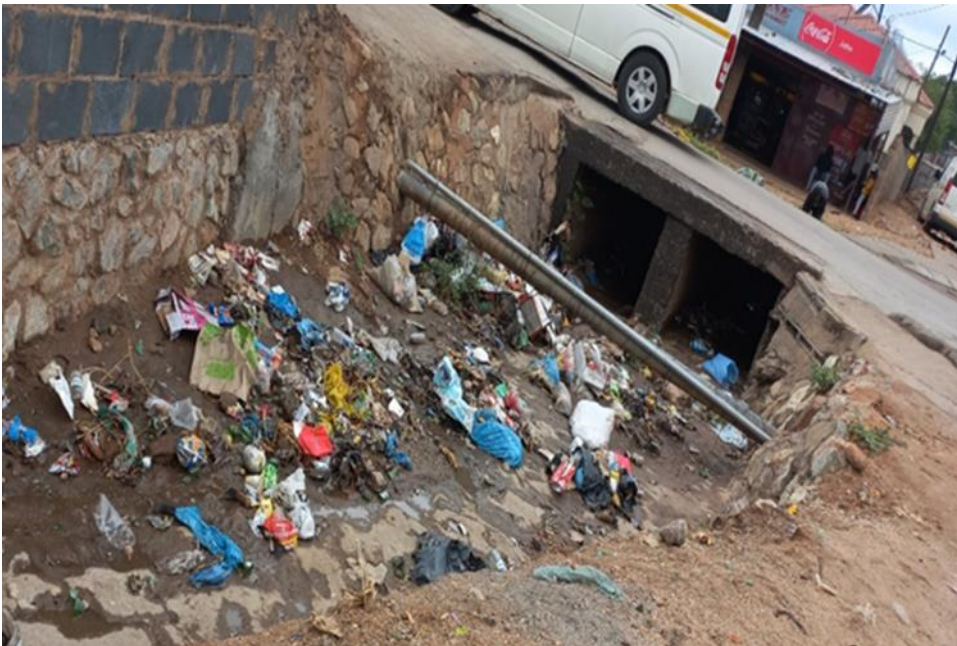
Figure 9: A Culvert in Musina
