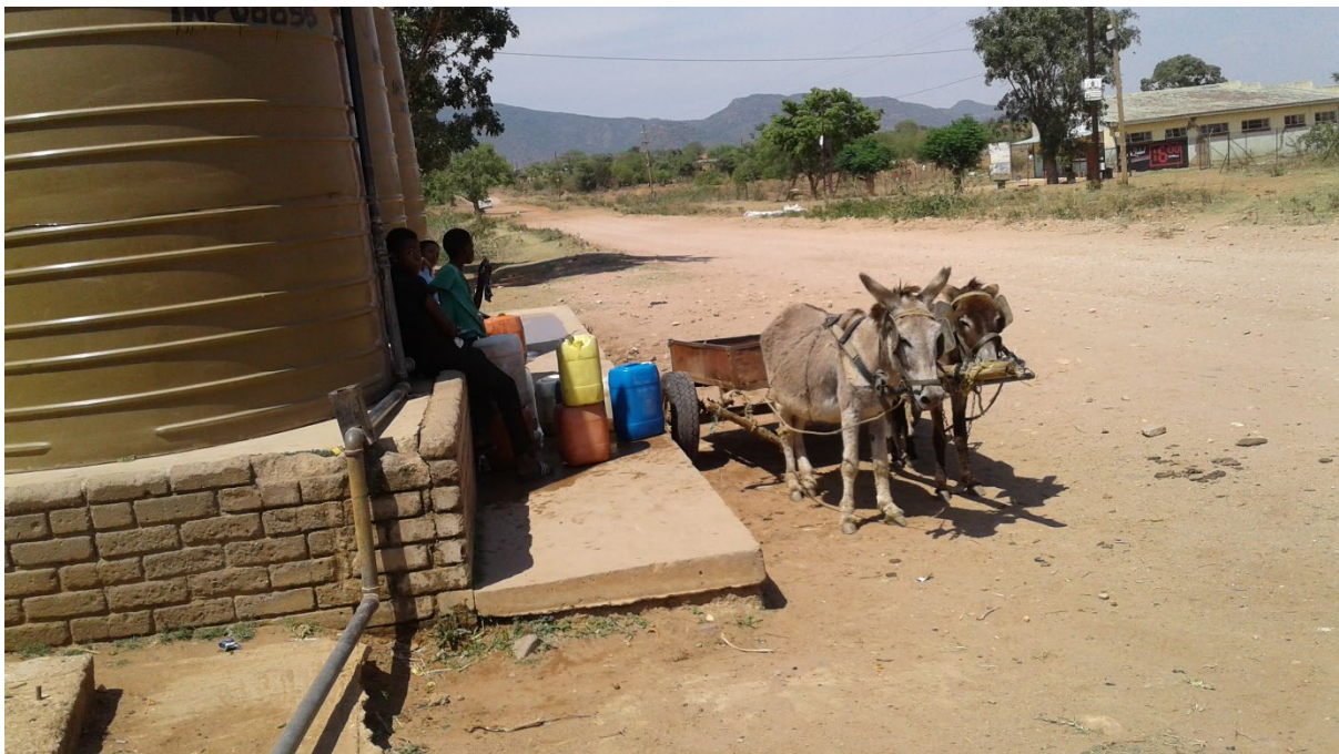
Picture 4. 14: Community street water tank
