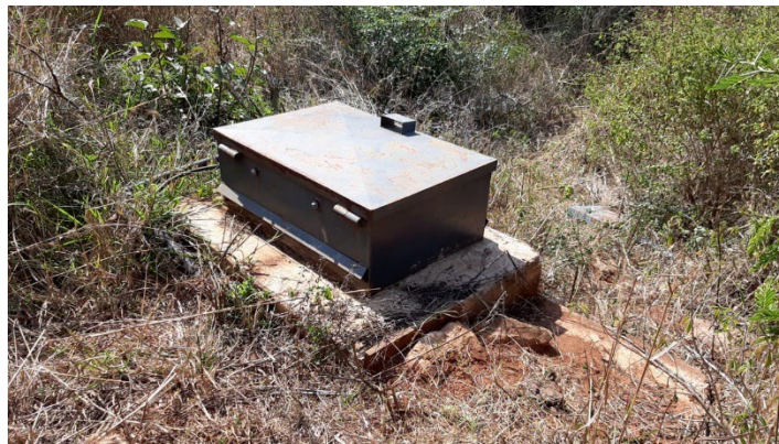
Plate 6: Existing Dzamba borehole (BH 3)
