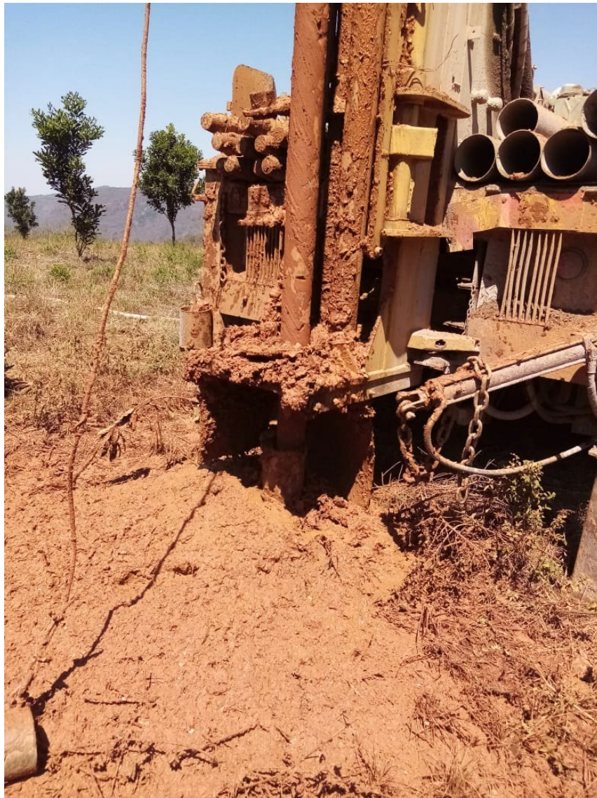
Figure 4-10: Mabulo Village Existing Borehole (B2) rehabilitation
