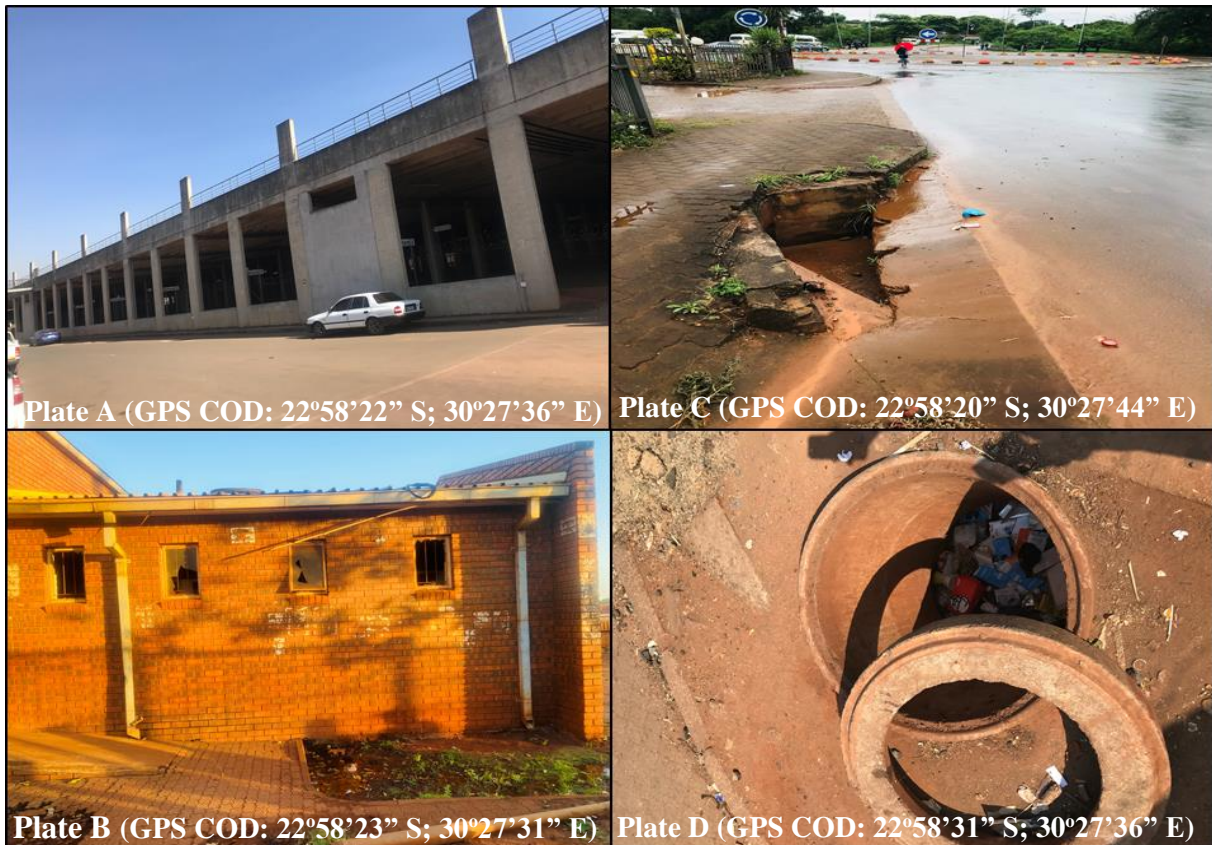
Photograph 5.3: Urban decay features related to collapsing infrastructure and abandoned projects in Thohoyandou Town CBD Source: Fieldwork (2023)
