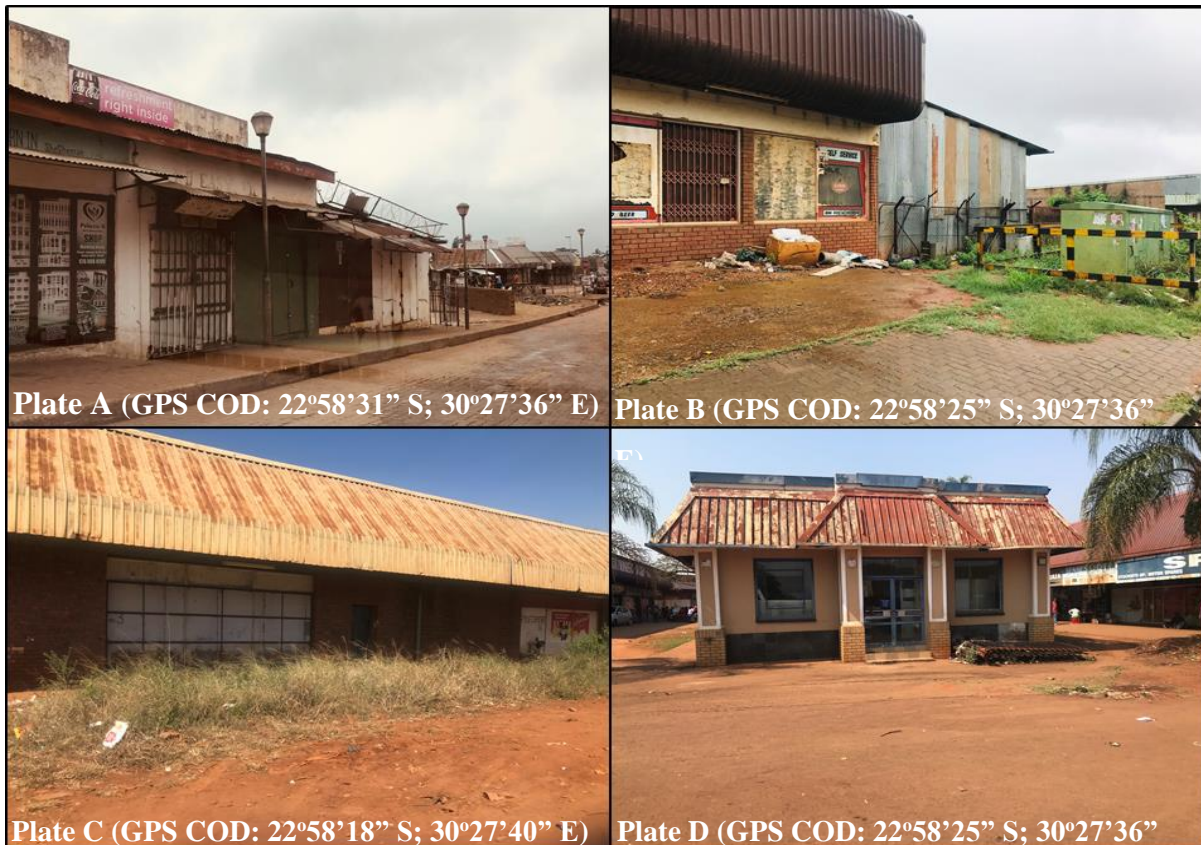
Photograph 5.4: Urban decay features related to collapsing infrastructure and abandoned projects in Thohoyandou Town CBD Source: Fieldwork (2023)
