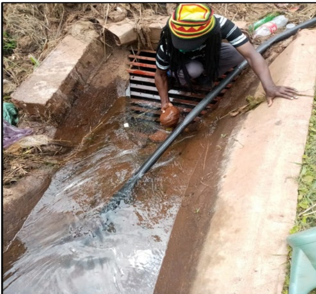
Figure 4.8: Offtake pipes and rocks for informal water abstraction
