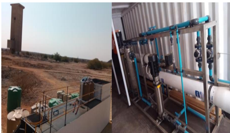
Figure 2.24: Water treatment pilot plant mobilisation
