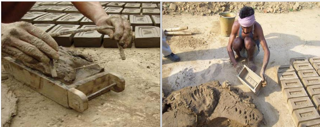
Figure 2.2: Placing the clay in a mould to form bricks (Mueller et al. , 2008)
