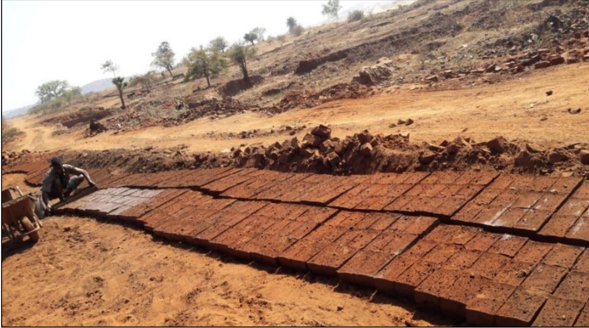
Figure 4.14: Material preparation and brick moulding in one of the selected areas in Dididi
