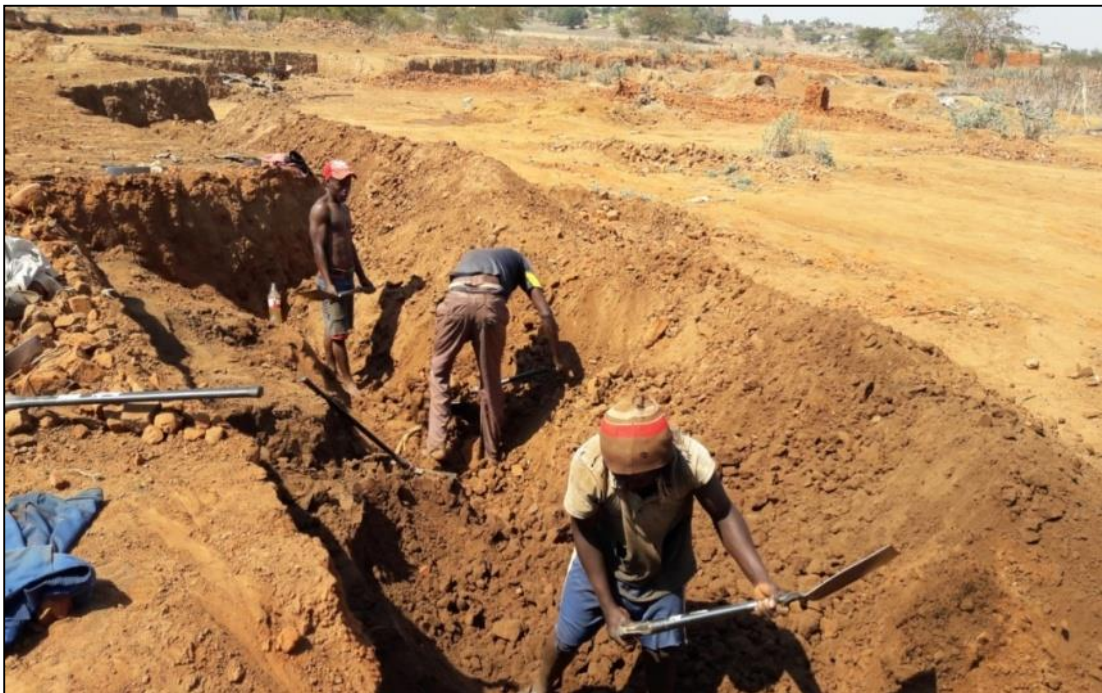
Figure 4.12: The operations of extraction of raw material for bricks manufacturing
