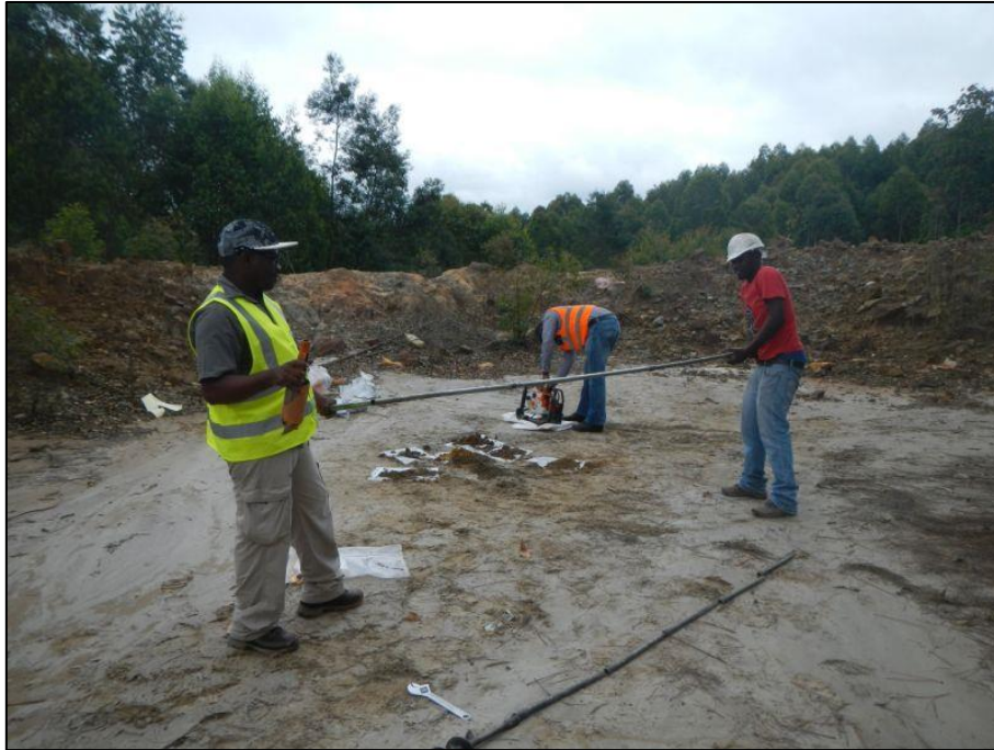
Figure 4 Two meters handheld auger in Nestor Mine tailings storage facility
