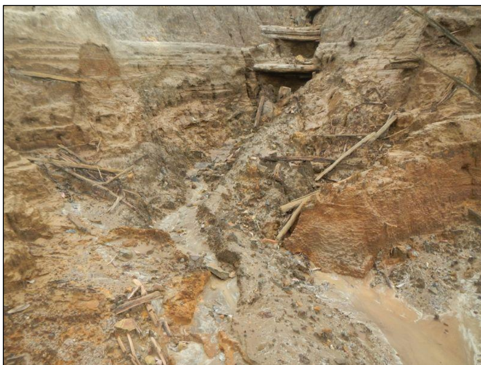
Figure 10 Weathered Nestor TSF
