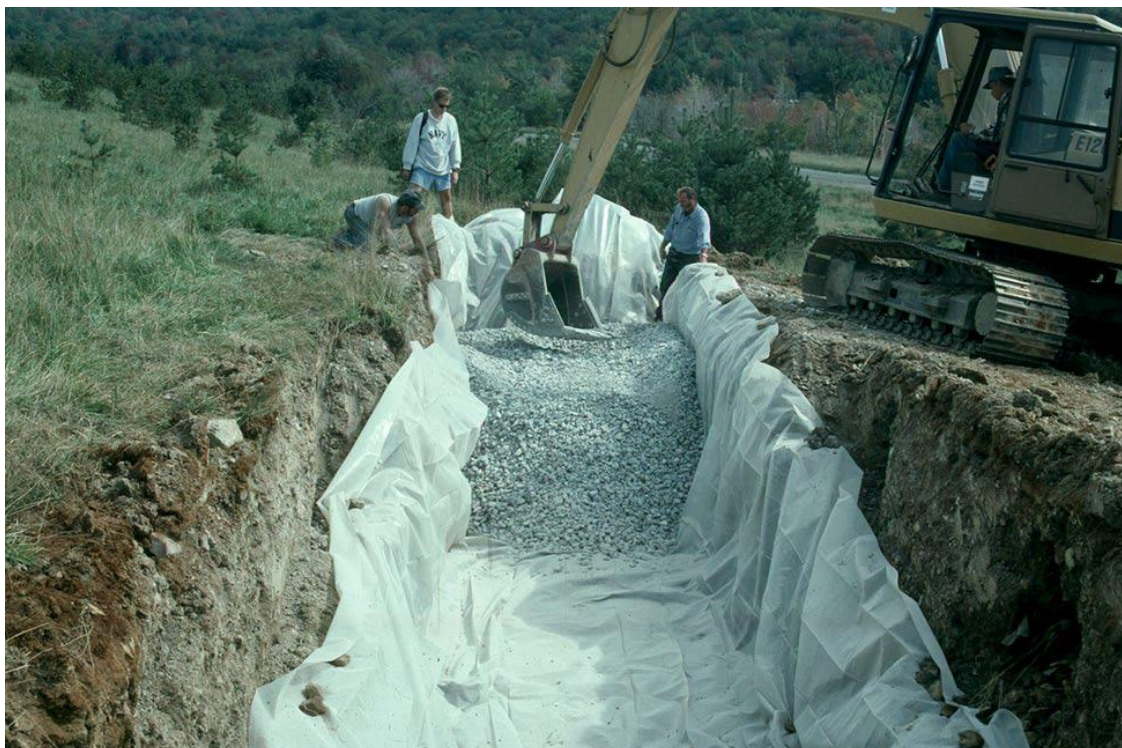
Figure 2. 3: Anoxic limestone drains (Skousen et al., 2017).
