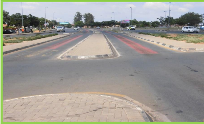
Plate 4.2. Illustrates a two-way median-aligned bus way in the T3 trunk route, where the BRT Rea-Vaya lanes are indicated through the red markings.
