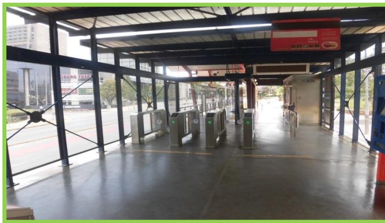
Plate 4.8. Safety enclosed and comfortable BRT Rea-Vaya station
