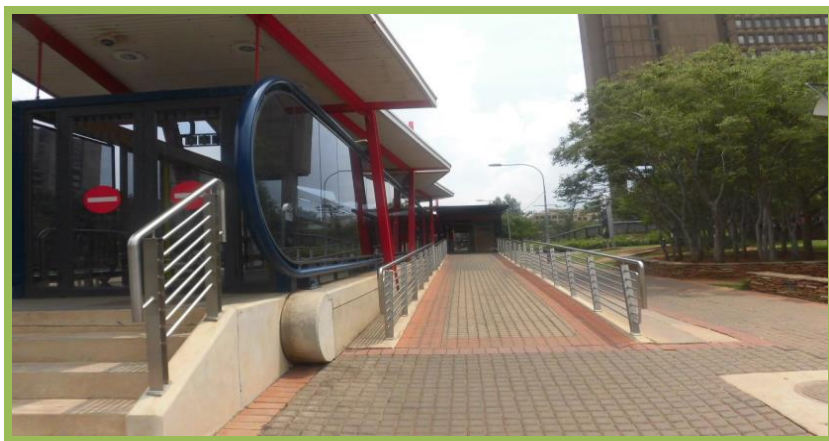
Plate 4.12 illustrates an elevated ramp designed to allow for easy access for physically impaired passengers at the Joburg Theatre station.
