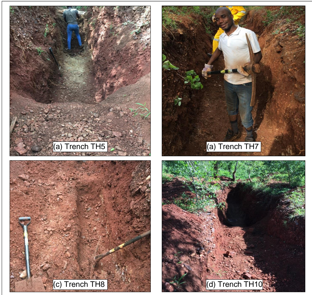
Figure 3.5: Manual excavation of trenches using pickaxe and shovel.
