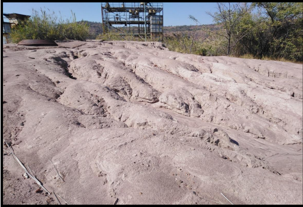
Figure 3.4: Heap A showing gully erosion.
