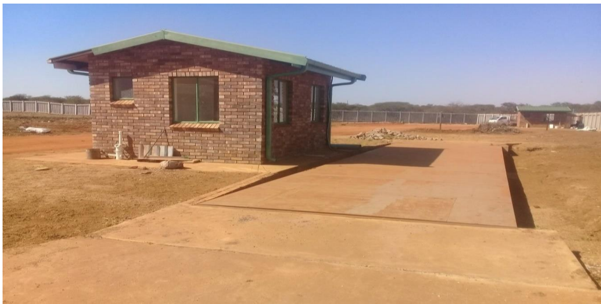
Figure 4. 30: Makhado Landfill site weighbridge.
