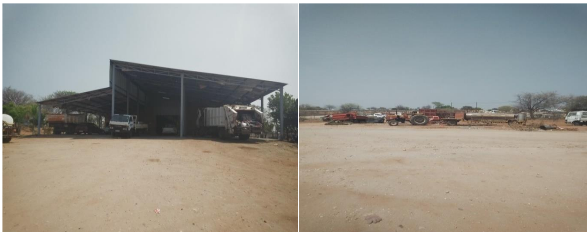
Figure 4. 44: Musina workshop facility for maintenance and repairing of equipment.
