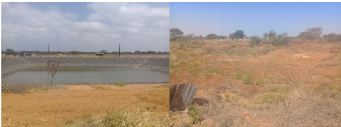
Figure 4. 42: Makhado and Thulamela Landfill site leachate ponds.
