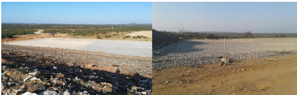
Figure 4. 40: Musina constructed disposal cell.
