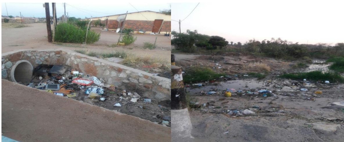
Figure 4. 49: Illegal dumping of waste in catchment areas in Musina Local Municipality.
