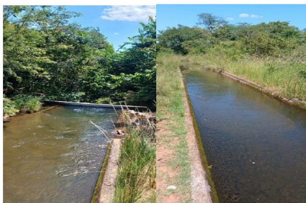
Figure 15: Main canal that transmits water from Mutale River to the Mbahela Irrigation Scheme
