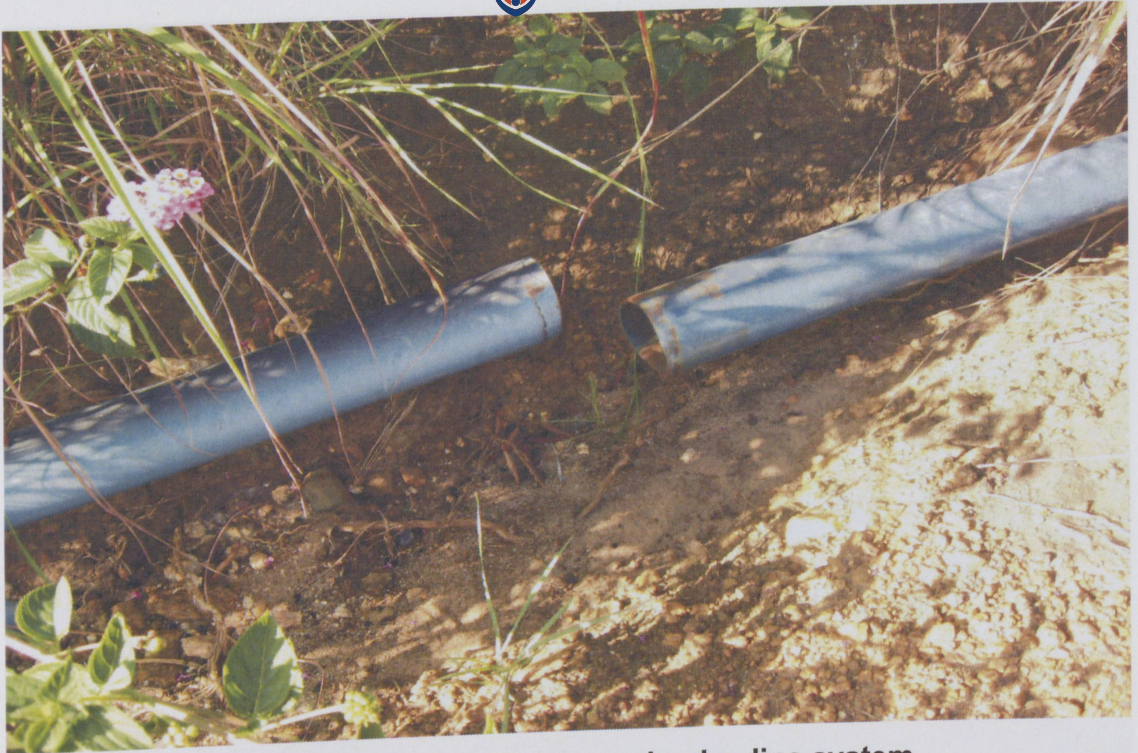
Picture 4.3: Breakdown and cut-off of the main pipe line system
