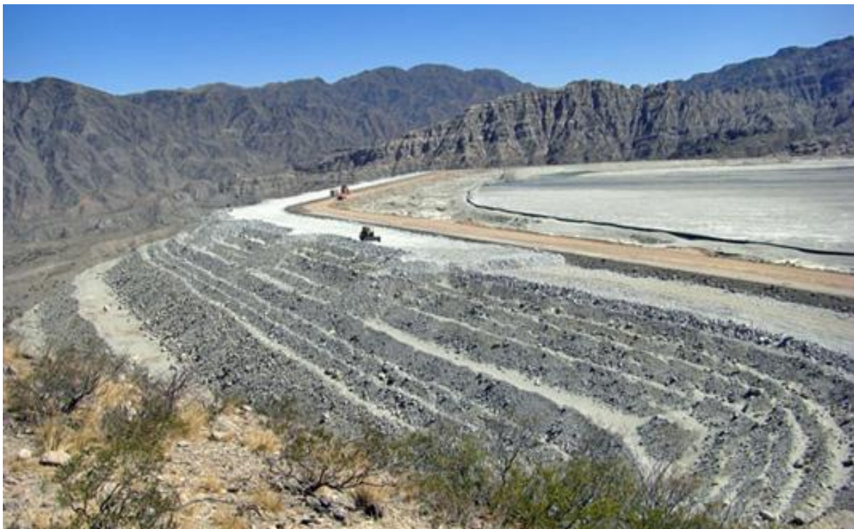
Figure 2.2: Shallow low velocity braided streams of subaerial technique of tailings deposition (Engels, 2006).
