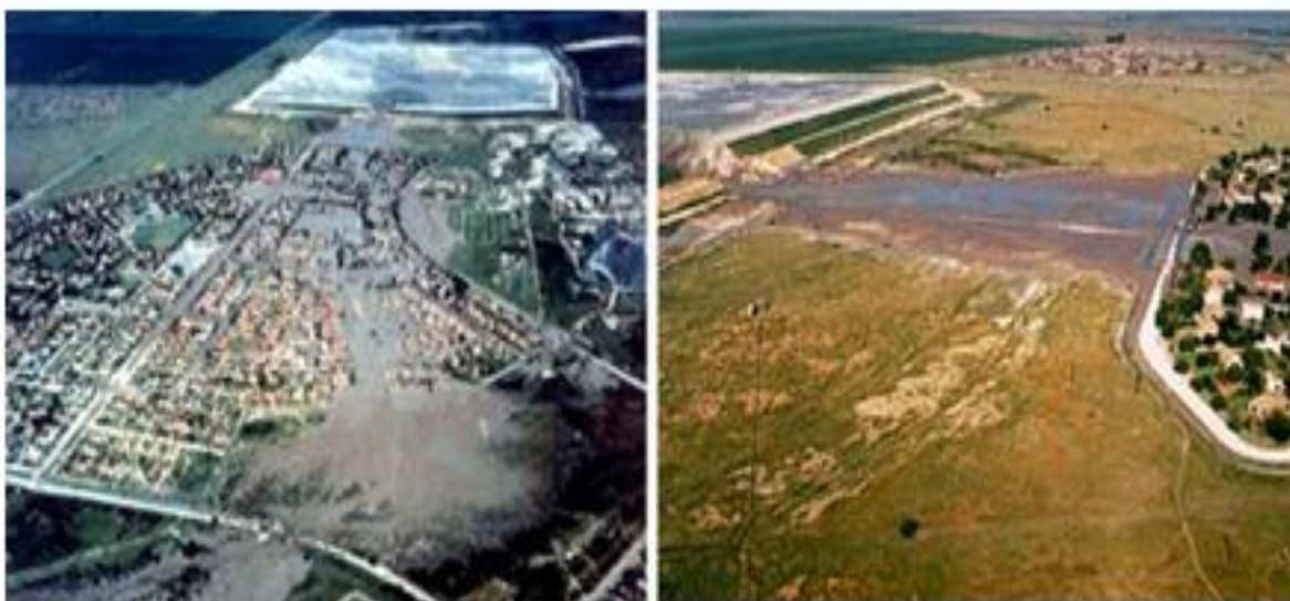
Figure 2.9: Marriespruit tailings dam failure in 1992 due to overtopping ( www.tailings.info/casestudies/marrespruit.html ).
