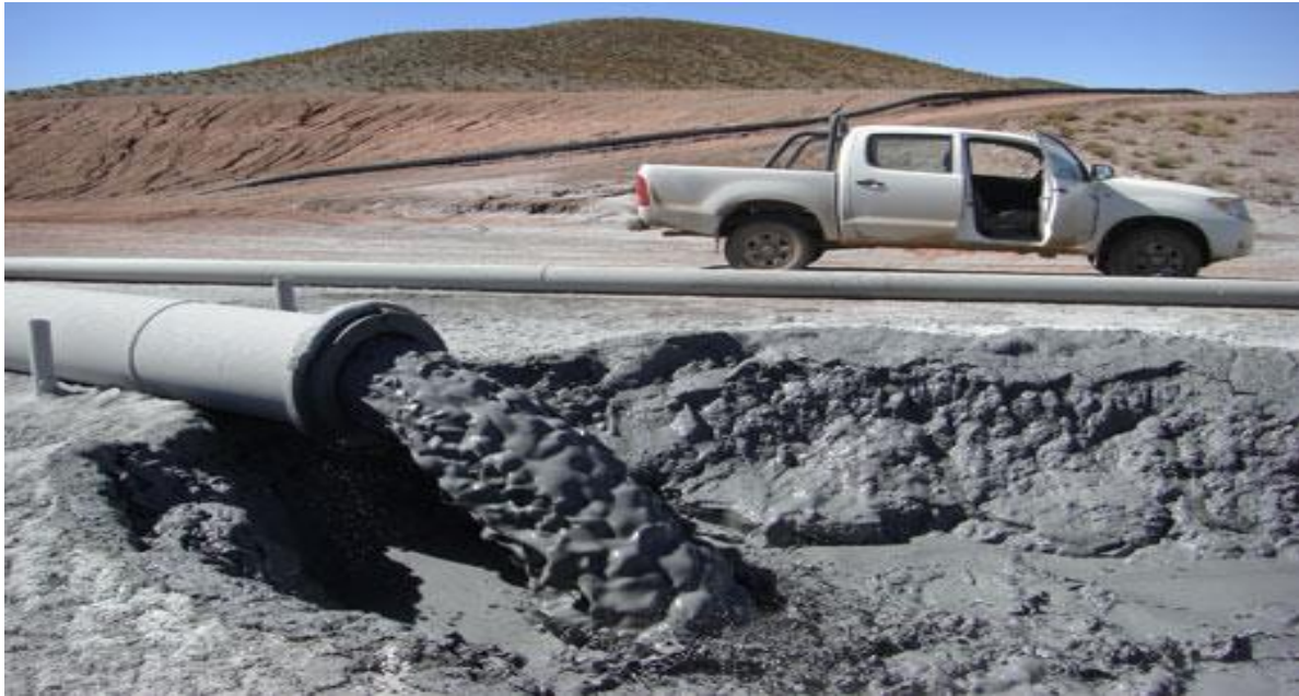
Figure 2.5: Large diameter pipe depositing tailings in single point technique of tailings deposition (Engels, 2006).
