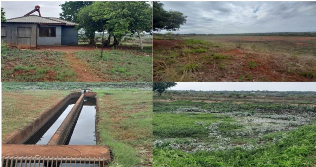
512 Figure 4.1: Images of a vandalized wastewater treatment pond facility with damaged buildings (top left), one dry 513 oxidation pond (top right), a functioning pre-treatment (bottom left) and a sparsely filled oxidation pond (bottom 514 right)
