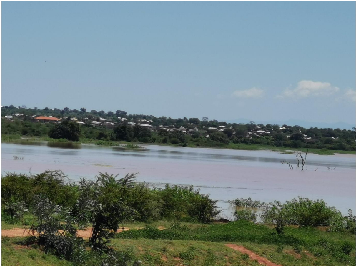
Figure 24: The Makuleke Dam (Source, Researcher, 2019)
