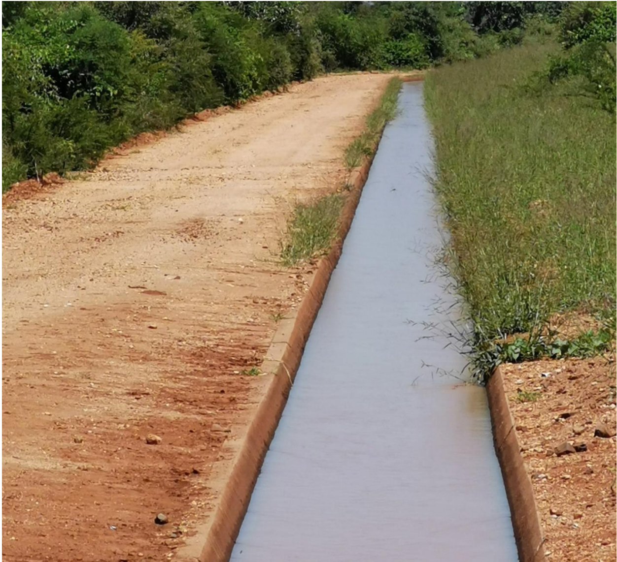
Figure 33: Makuleke canal from Makuleke Dam to Food Plots and Irrigation Scheme. (Photo, Researcher, 2020)
