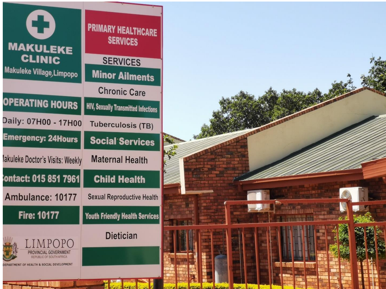
Figure 40: The Makuleke Clinic. Built by the CPA. (Photo, Researcher, 2020)
