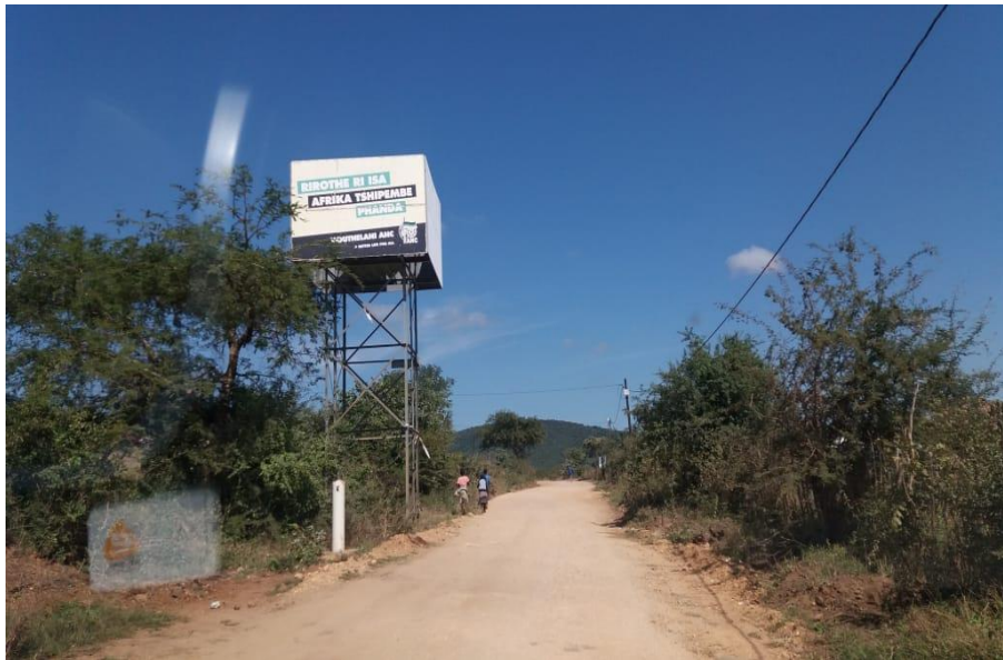
Figure 6.6 Water Tanks in the Village
