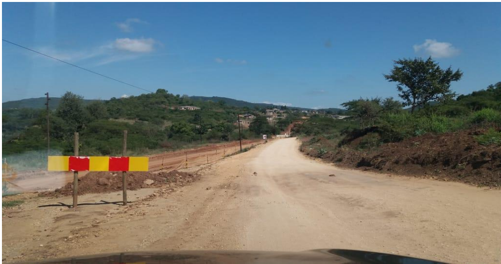
Figure 6.7 Construction of a Tarmac Road in the Village
