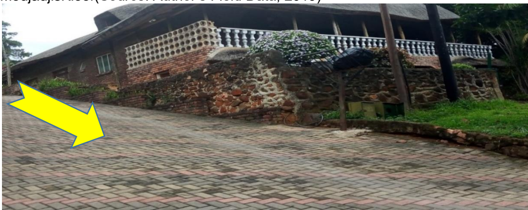
Plate 5.8: impervious surfacing as adaptation strategy against threats caused by steep elevation in Modjadjiskloof (Source Author's Field Data, 2019)
