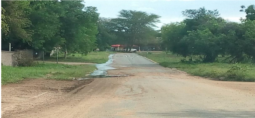
Plate 5.9: The impact of surface runoff in the absence of drainages on Hans Pirow Lu Street inPhalaborwa (Source: Author's Field Photo, 2019)
