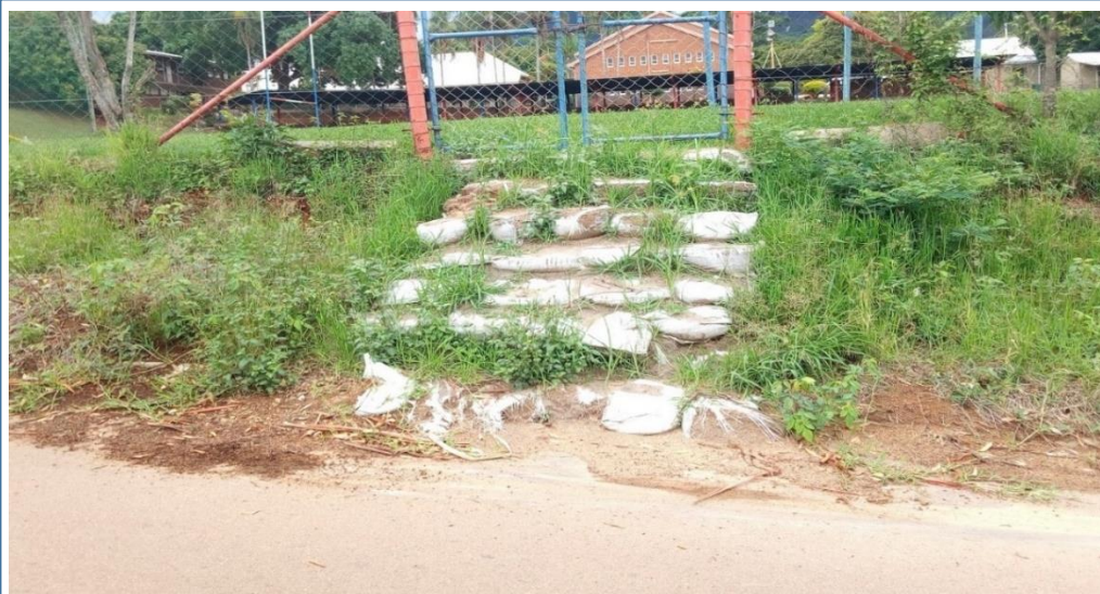
Plate 7.5: Use of sandbags to protect properties against flooding (Source: Author's Field Photo, 2019)
