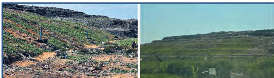
Figure 2: Bench with gas release pipes.
