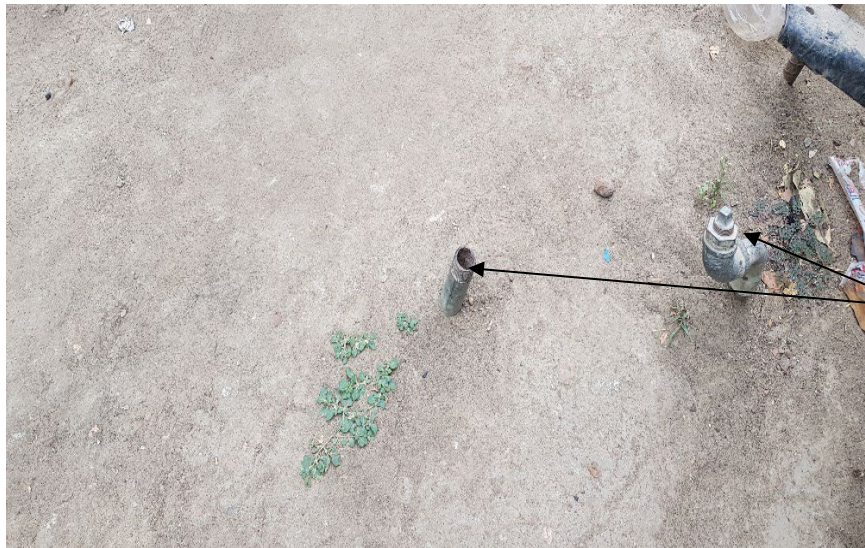
Figure 6.26: A disconnected water supply system in Runyararo West high density suburb of the City of Masvingo
