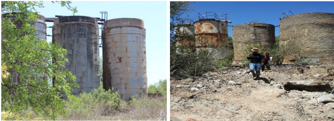
Figure 4. 7: Abandoned silos and excavations by artisanal miners around these structures
