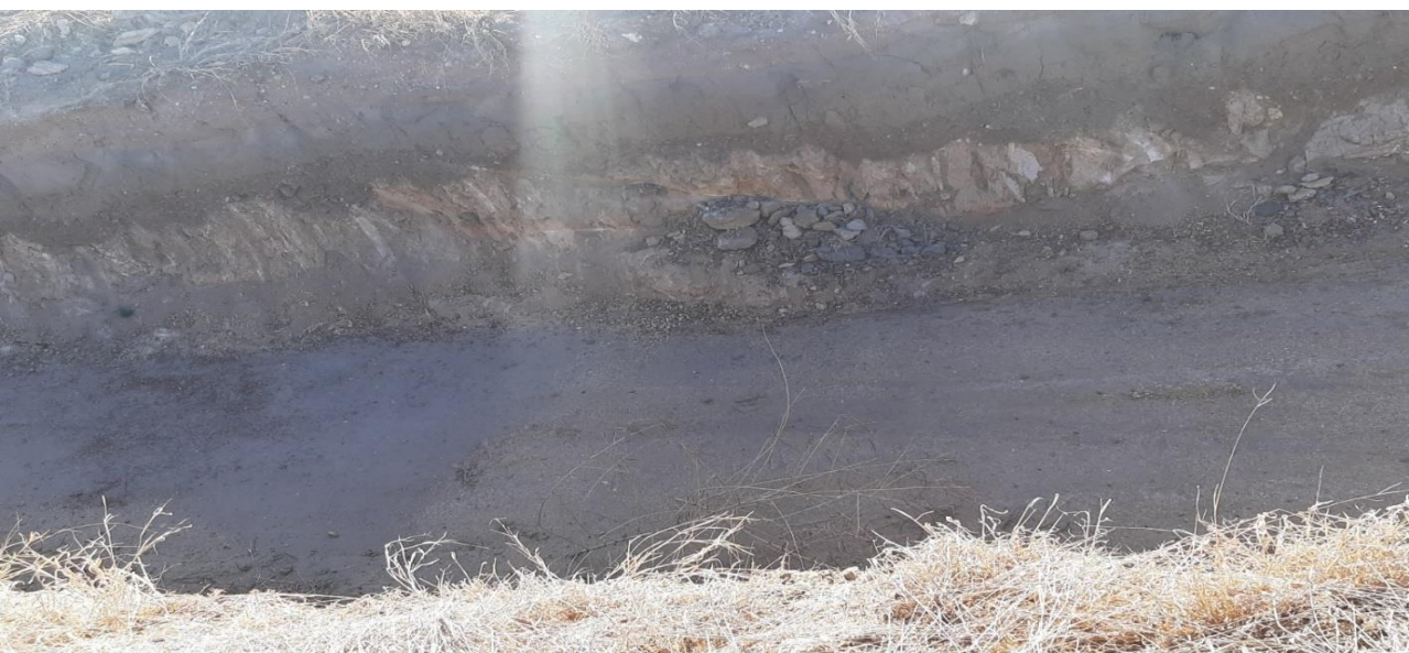
Figure 6.9: Incorrect water pipelines exhumed, and trench left bare
