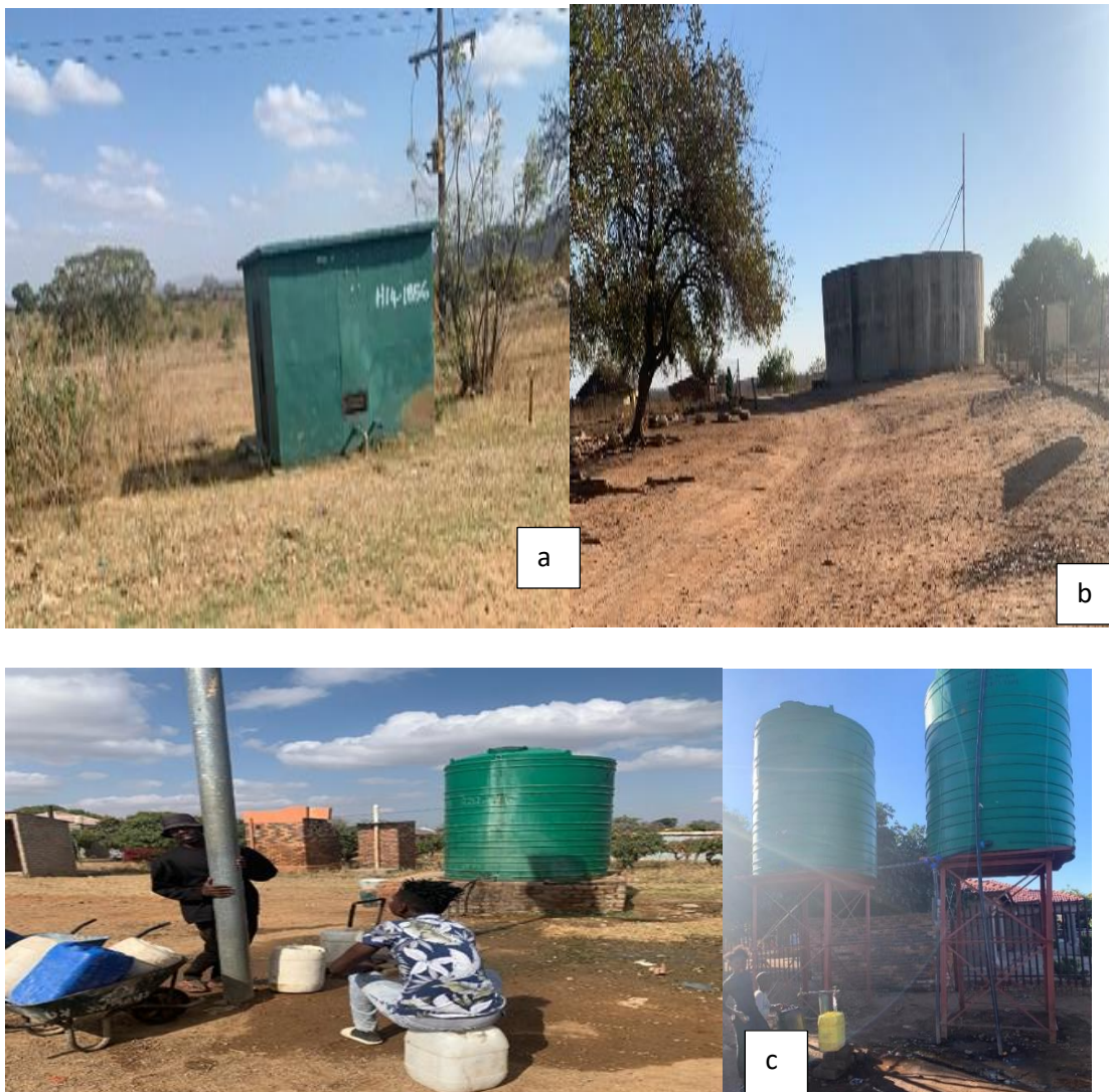
Figure 4.1: Borehole water supply in the study area, (a) Municipal borehole (b) Reservoir storage and (c) JoJo tanks storage
