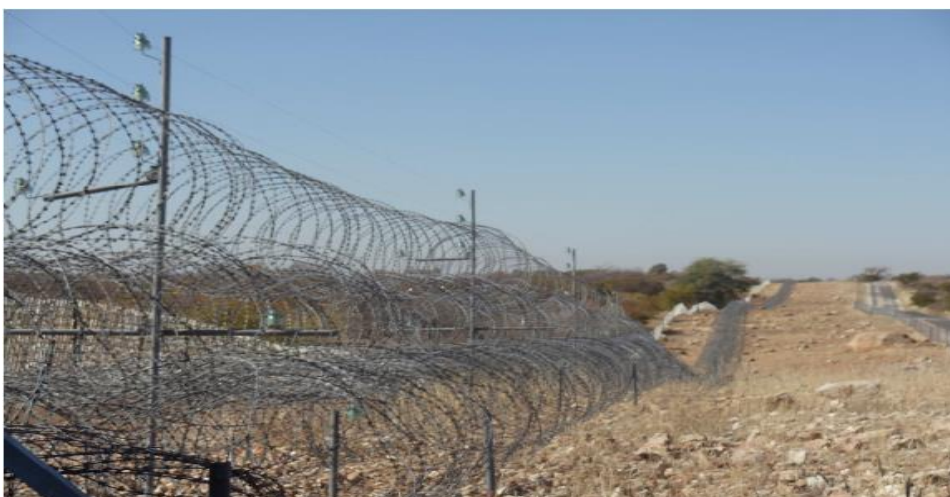
Figure 1: The triple layer of razor sharp wire barrier in the no man's land.
