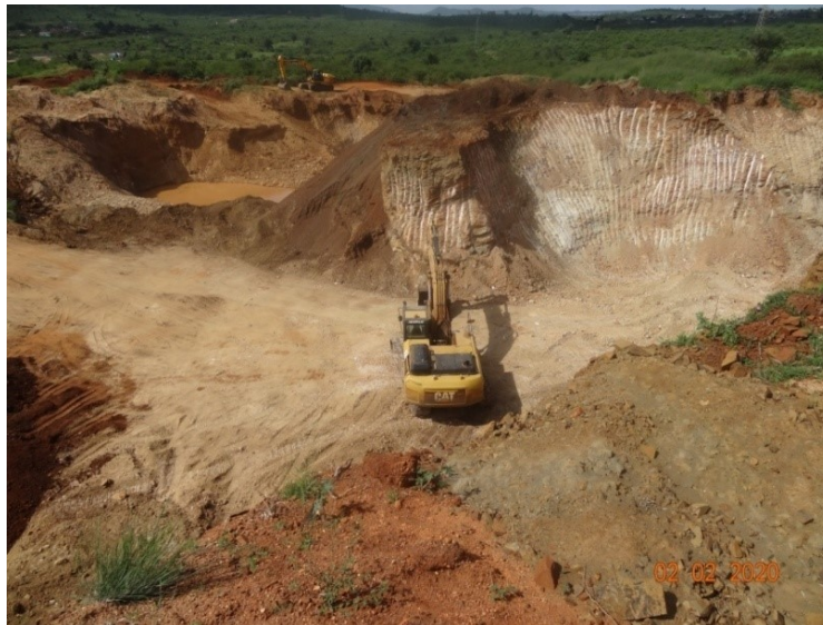
Figure 4.2: Excavators at gravel mining operation
