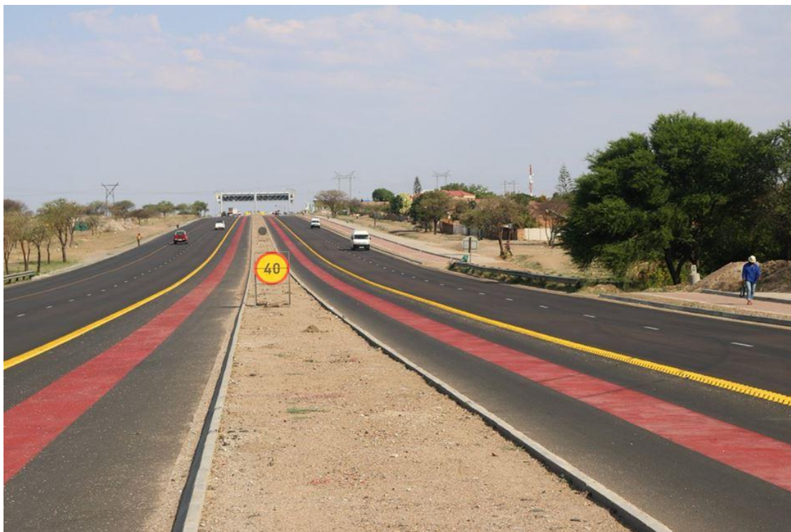
Plate 7.2: Nelson Mandela Drive spatial transformation to Leeto la Polokwane BRT system
