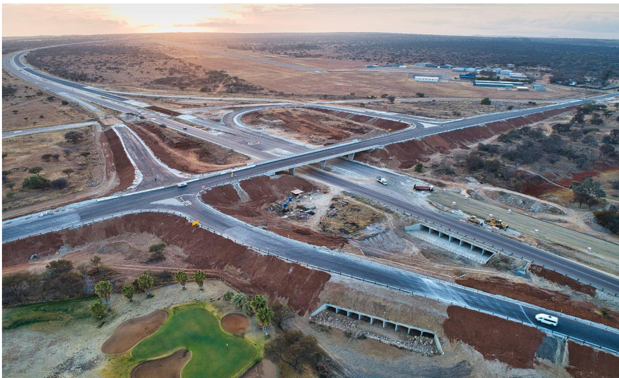
Plate 7.1: Polokwane N1 Eastern by-pass road structural spatial transformation
