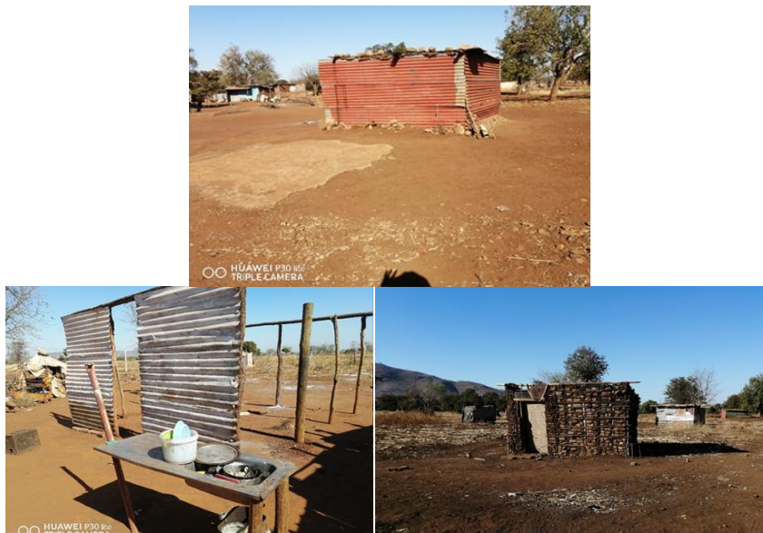
Photograph 6.1. Shacks destroyed due to winds and floods
