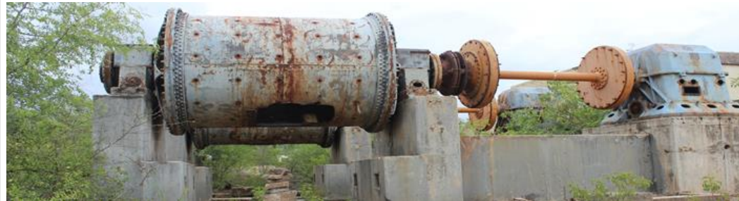
Mineral processing plant at Klein Letaba Mine
