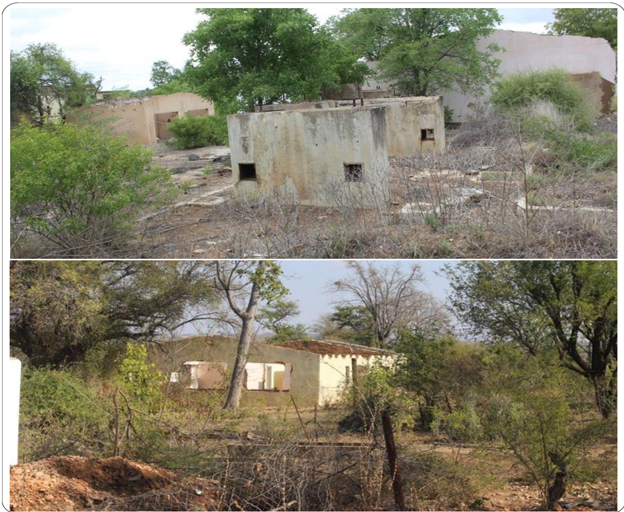
Figure 4.9: An illustration of vandalized abandoned building at Klein Letaba Mine.
