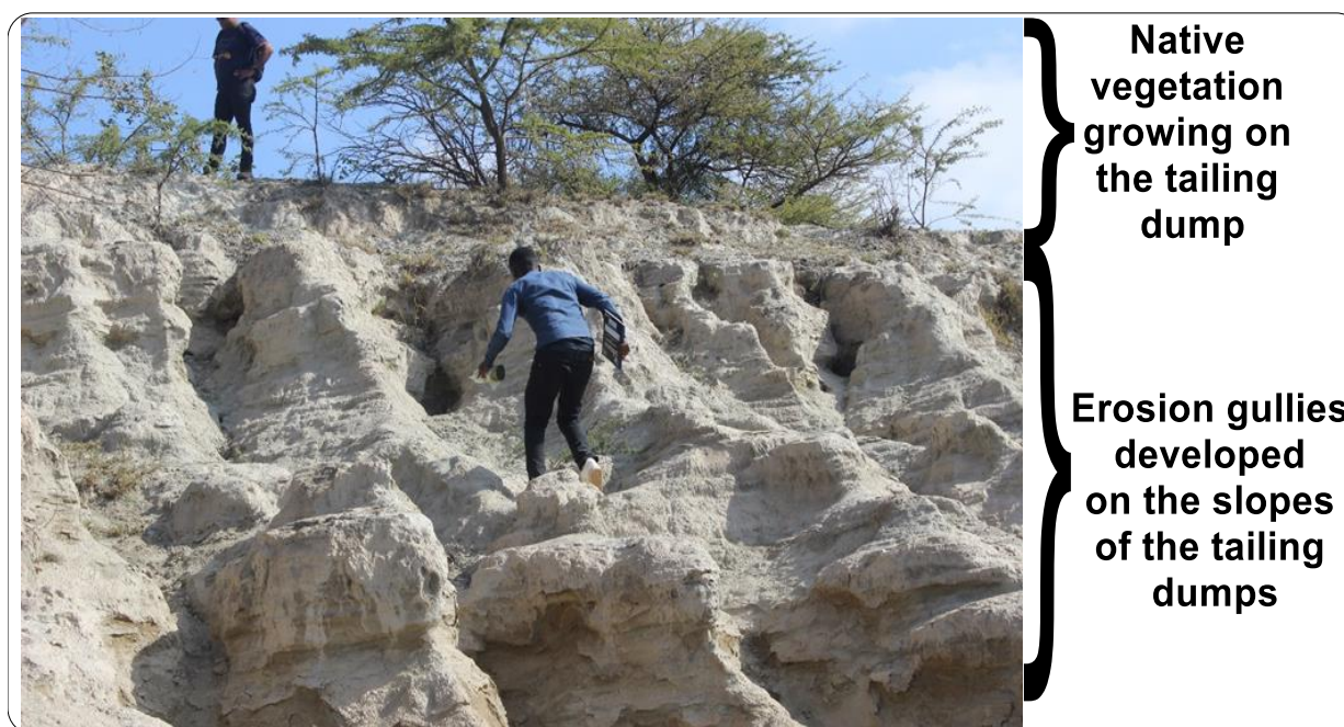
Figure 4.6: Evidence of growth of vegetation on the top surface and devastating effects of gully erosion on the slope of tailings.
