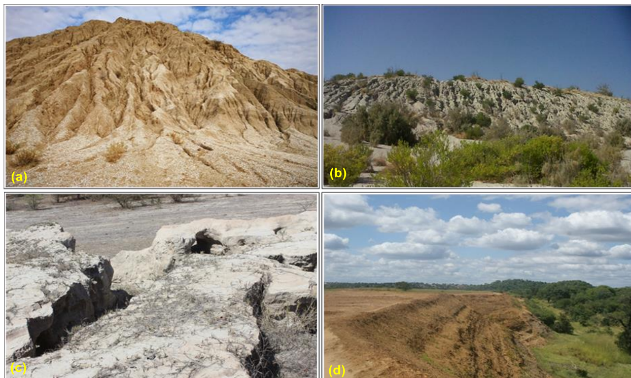
Figure 4.8: Illustration of the devastating effect of erosion on the slopes of tailings dumps. (a) is magnesite tailing, (b) is copper tailings dumps, (c) is the nature of piping erosion on Louis Moore mine tailings and (d) show the stable slopes of Klein Letaba gold mine tailings.
