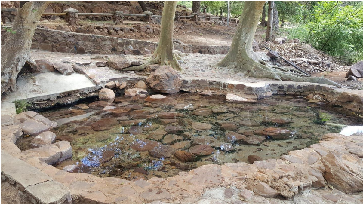
Figure 2.2 Mphephu thermal spring reservoir.
