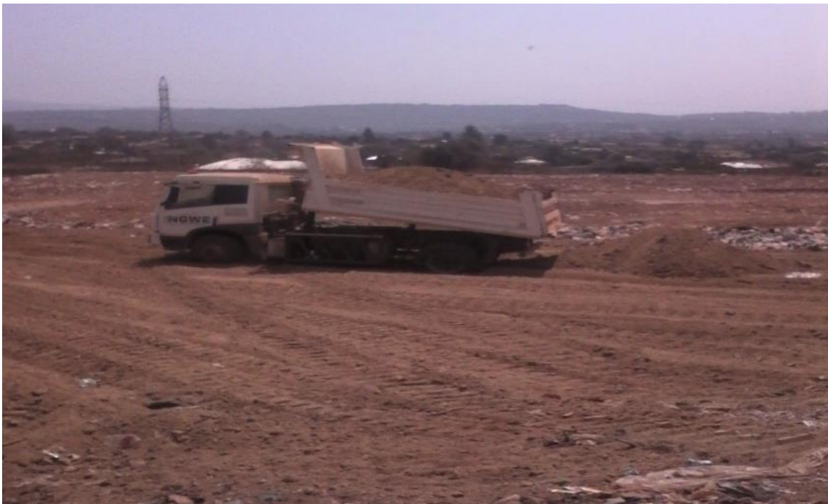
Figure 4.6: Tipper truck unloading soil for covering
