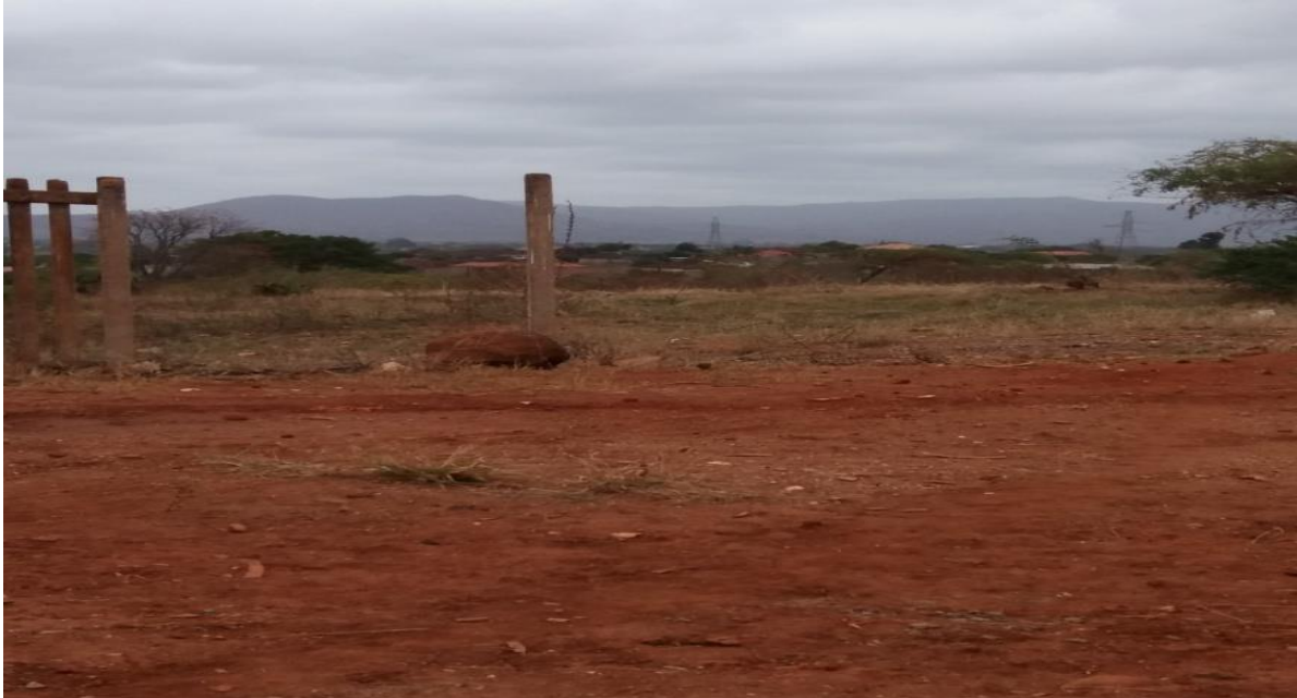
Figure 4.9: The TBJ landfill site's damaged fence
