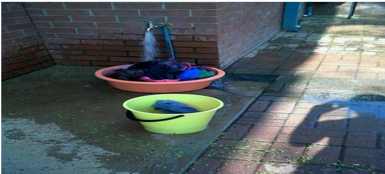
Figure 4.15: Water wastage at students residences
