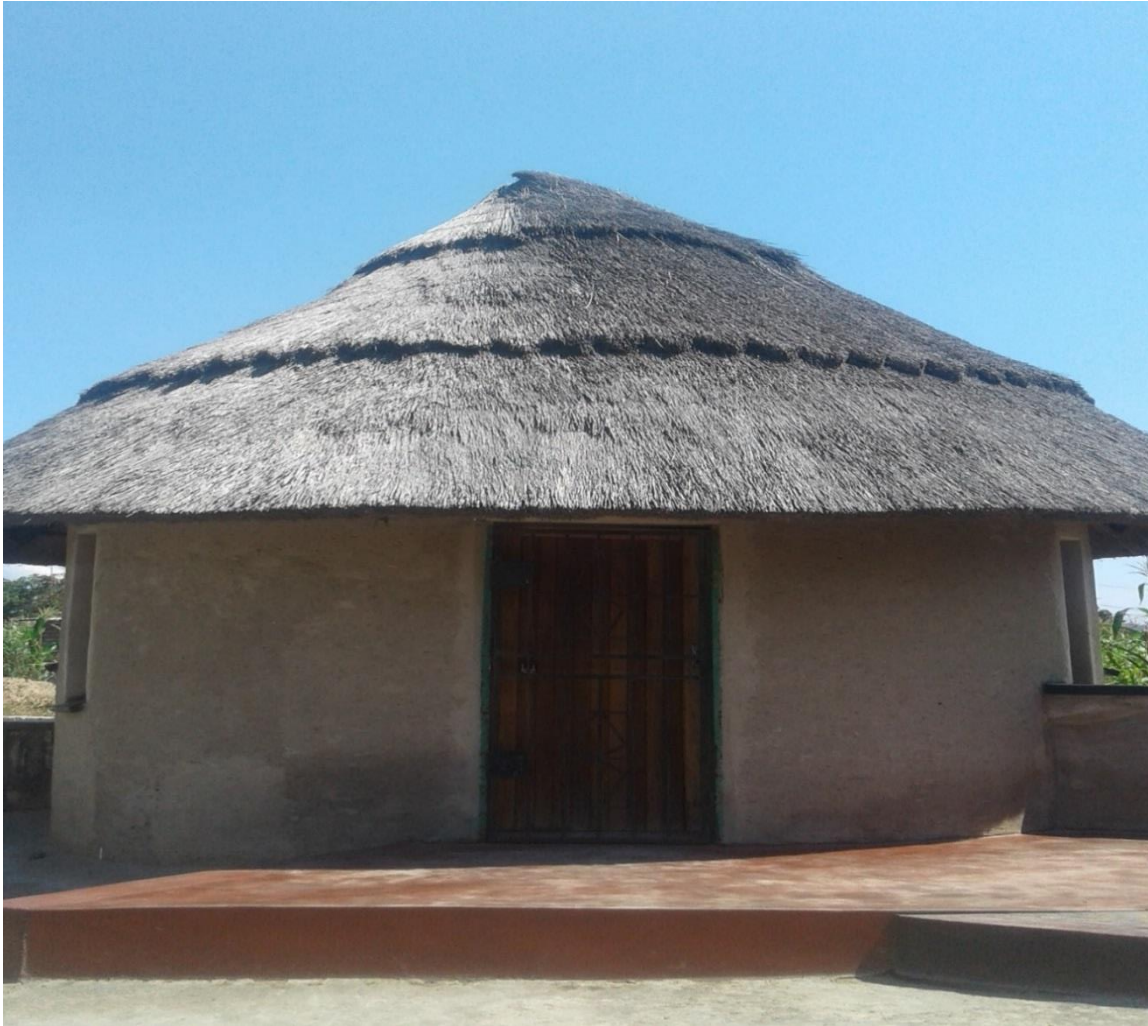
Figure 13. Stepped style decorative roofing on hut at Tšhabelang Village within the Greater Letaba municipality of Mopani District, Limpopo (March 23, 2017).
