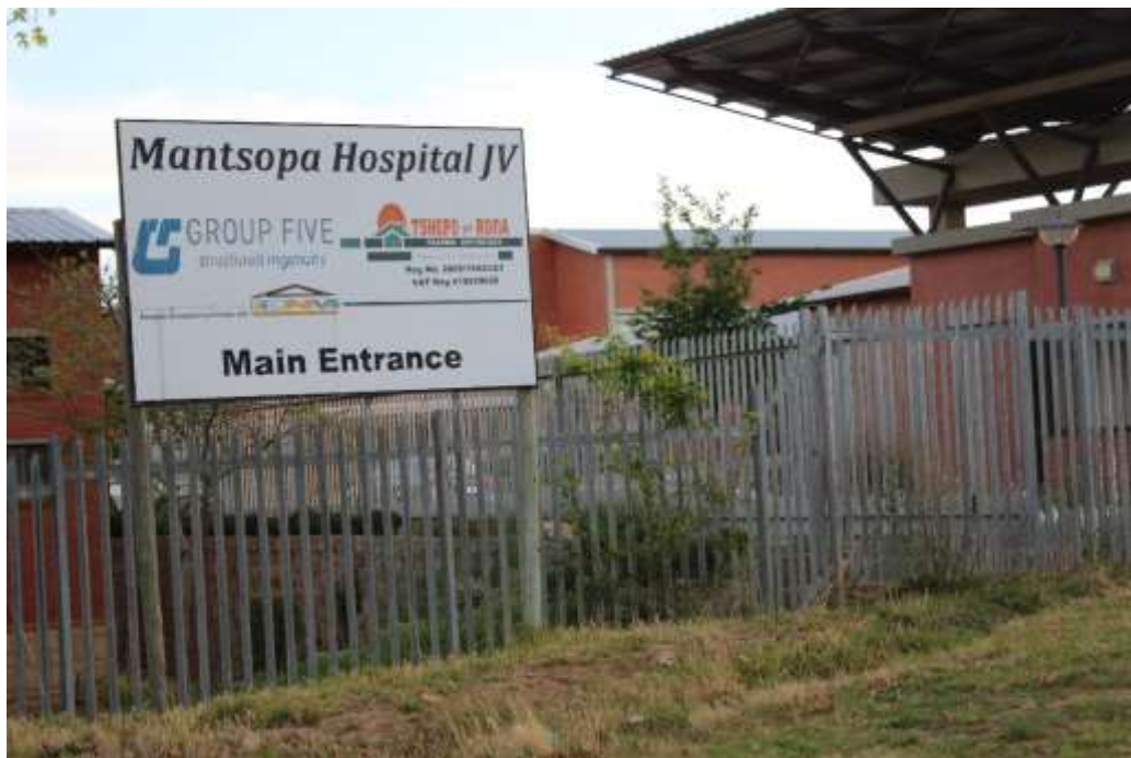
5.20 Image of New constructed Mantsopa Hospital JV by DHD Ngobese, 12/ 10/ 2017
